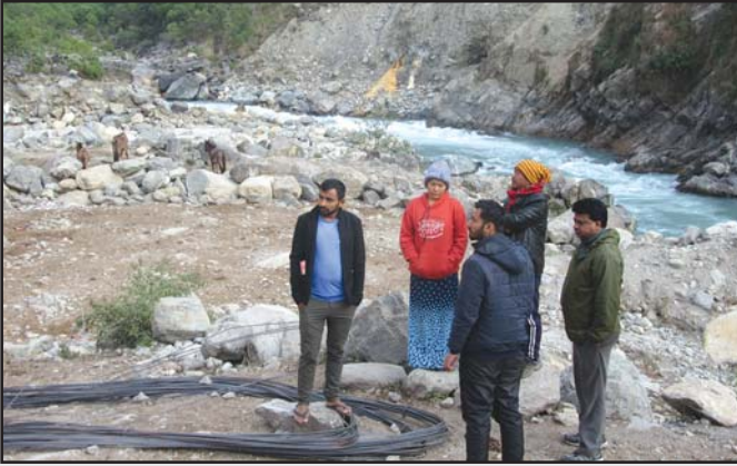
Site observation by government stakeholder to build rescue shelter, Gorkha
